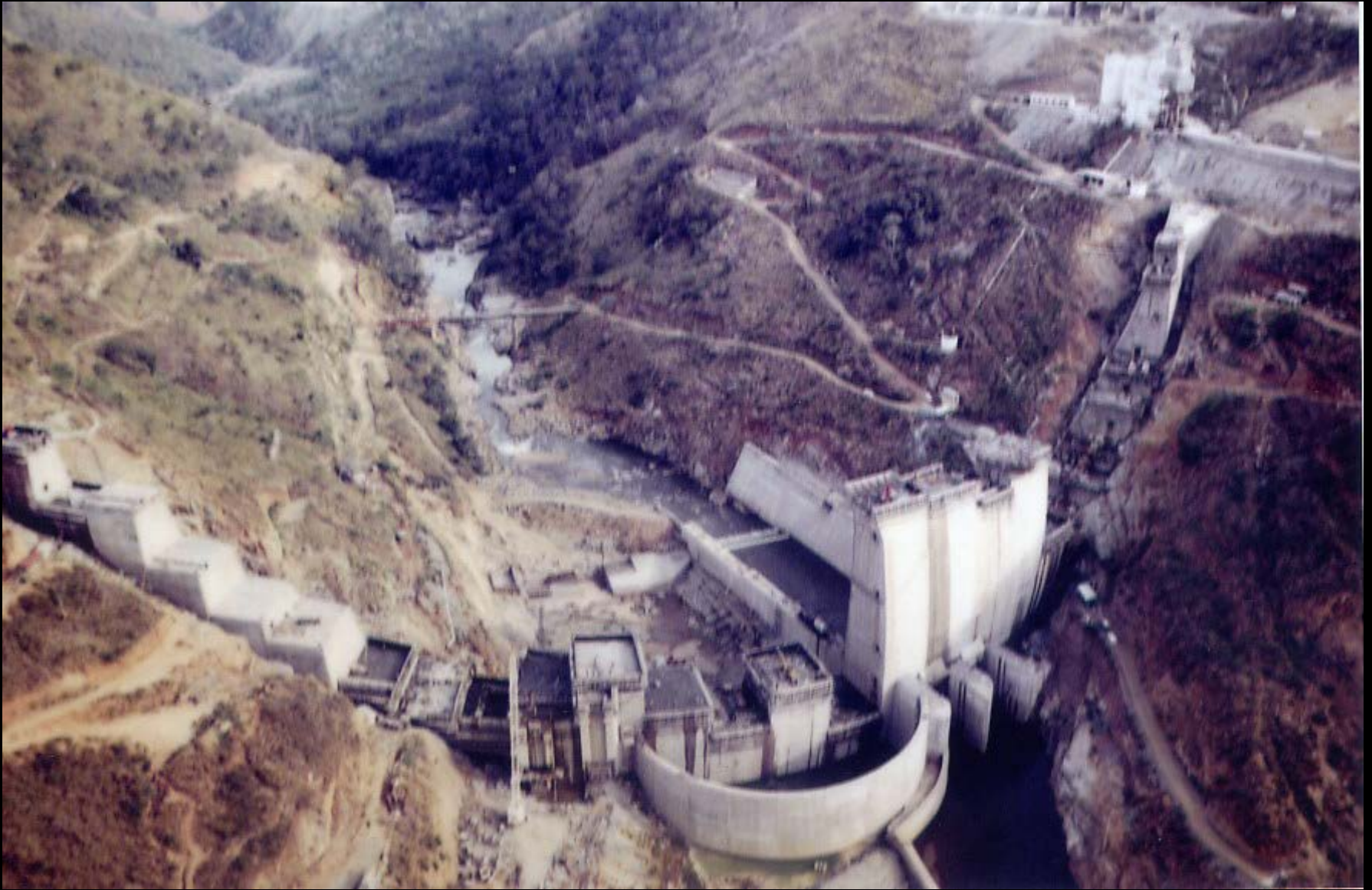
Dam Under Construction
